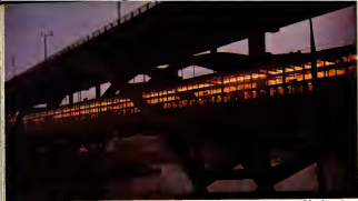
The station over the water: Lenin Hills station on bridge over Moskva river.
